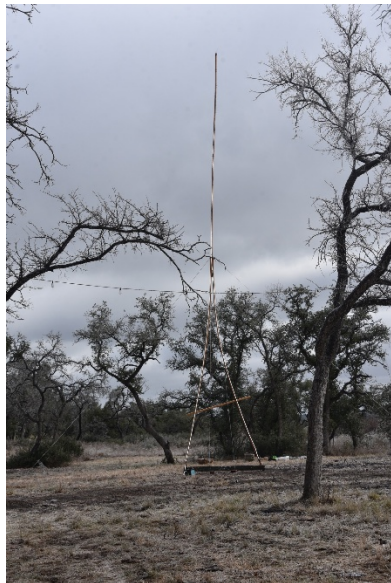
The vertical antenna was supported by a wooden tripod. Tim and the crew called it the "Awful Tower." It worked well and stood up to the wind and freezing rain. Tim said the horizontal loop he set up for 160m fell. I'm guessing it was from the weight of the built-up ice loading and wind.
