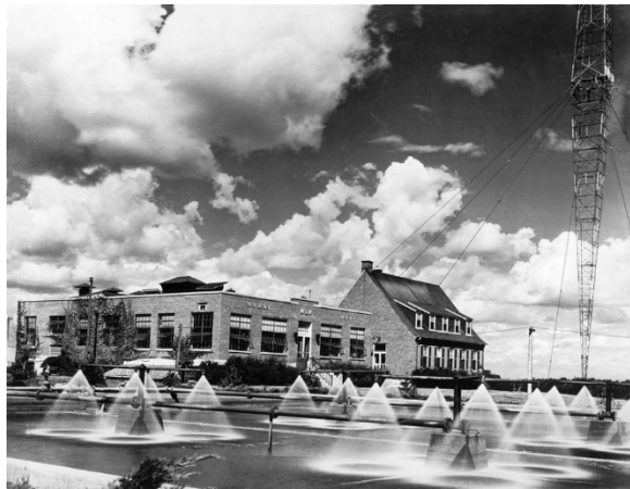
The 1934 500KW plant. Note the cooling pond with sprayers for cooling the transmitter (from thheRadio Historian)
