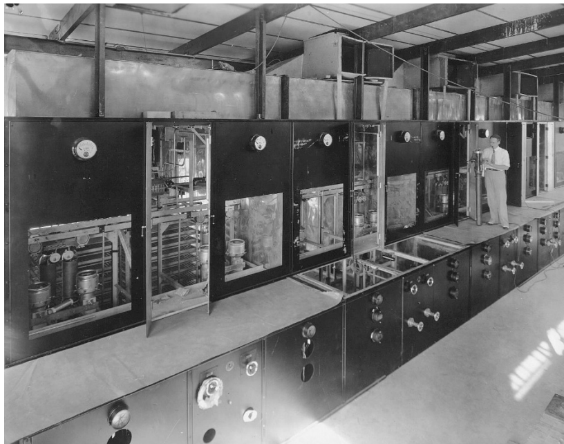
The 500KW transmitter during installation (from The Radio Historian)
