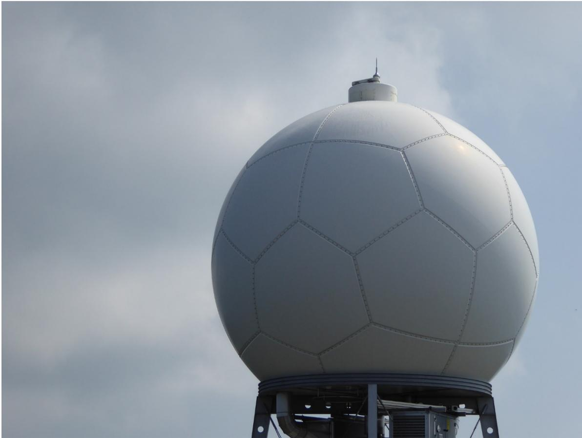
Doppler radar uses the Doppler effect to generate velocity data about things that are at a distance. As a microwave signal bounces off of the target, Doppler radar analyzes how motion alters the frequency of the returning signal. The difference provides an accurate measurement of the target's radial component velocity as it relates to the radar. Doppler radar is used in aviation, radio, police radar guns, health care (including radiology), meteorology, and even in Major League Baseball.
